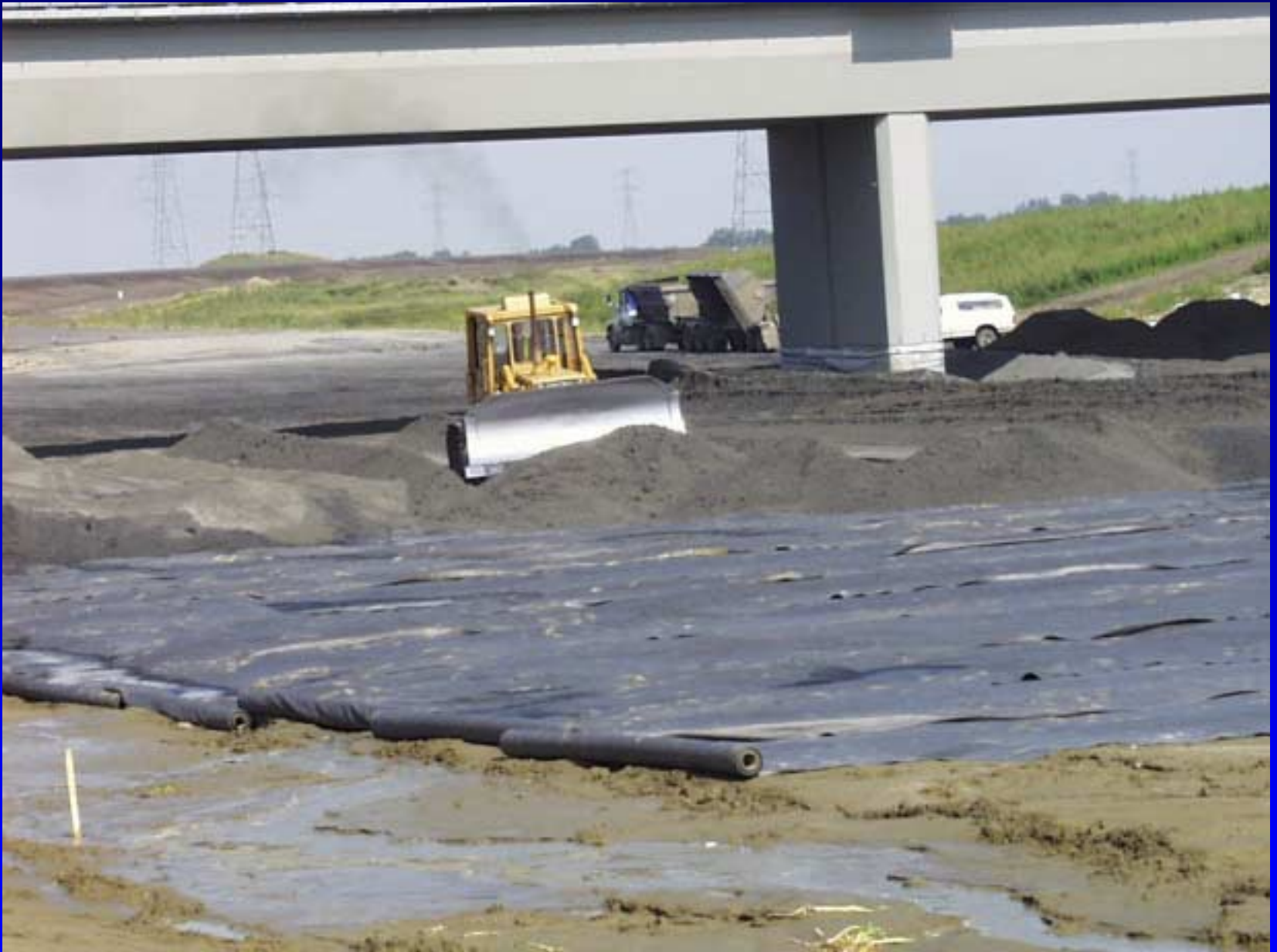
Bottom Ash Installation - Edmonton, Alberta
