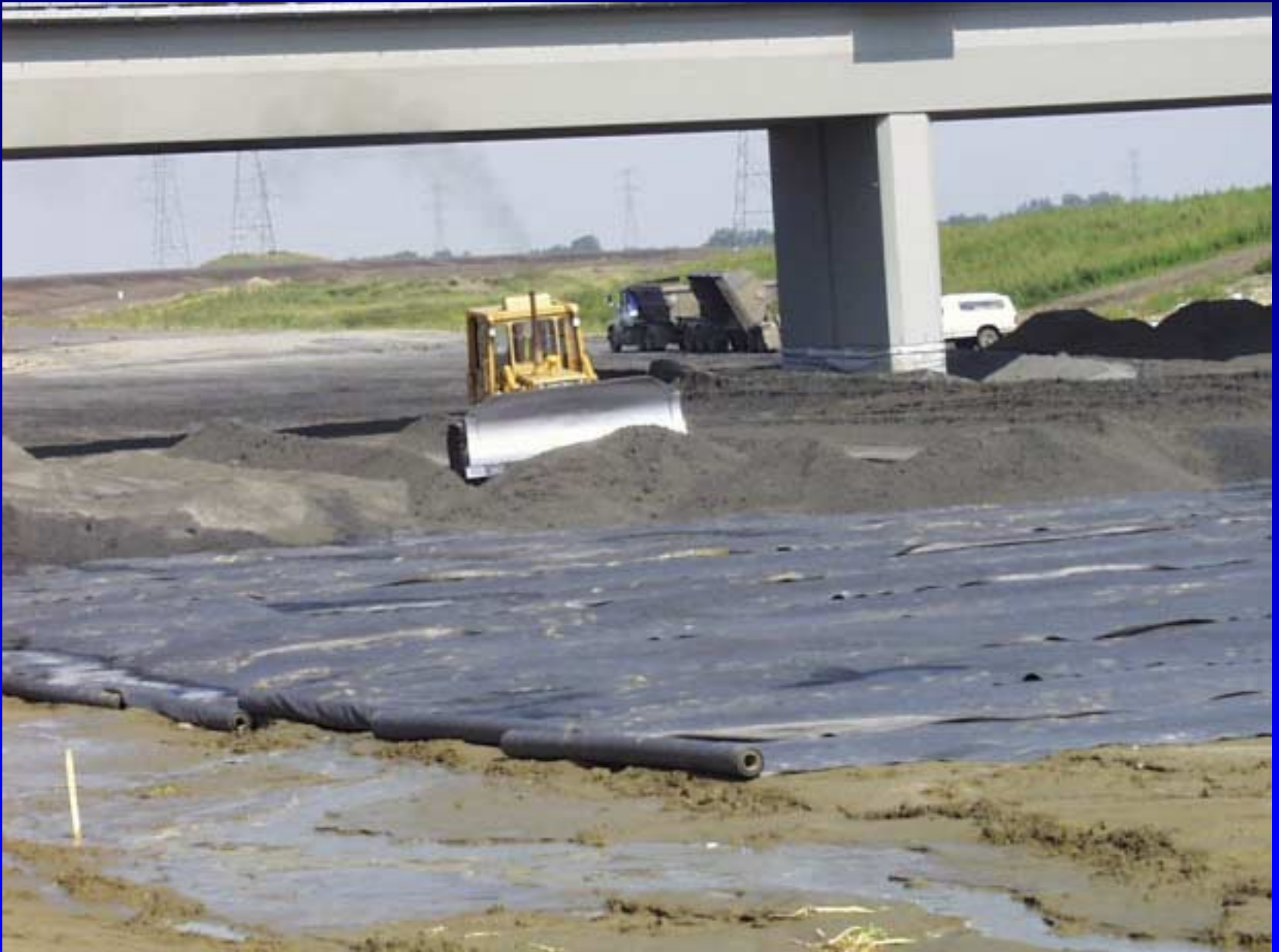
Bottom Ash Installation - Edmonton, Alberta
