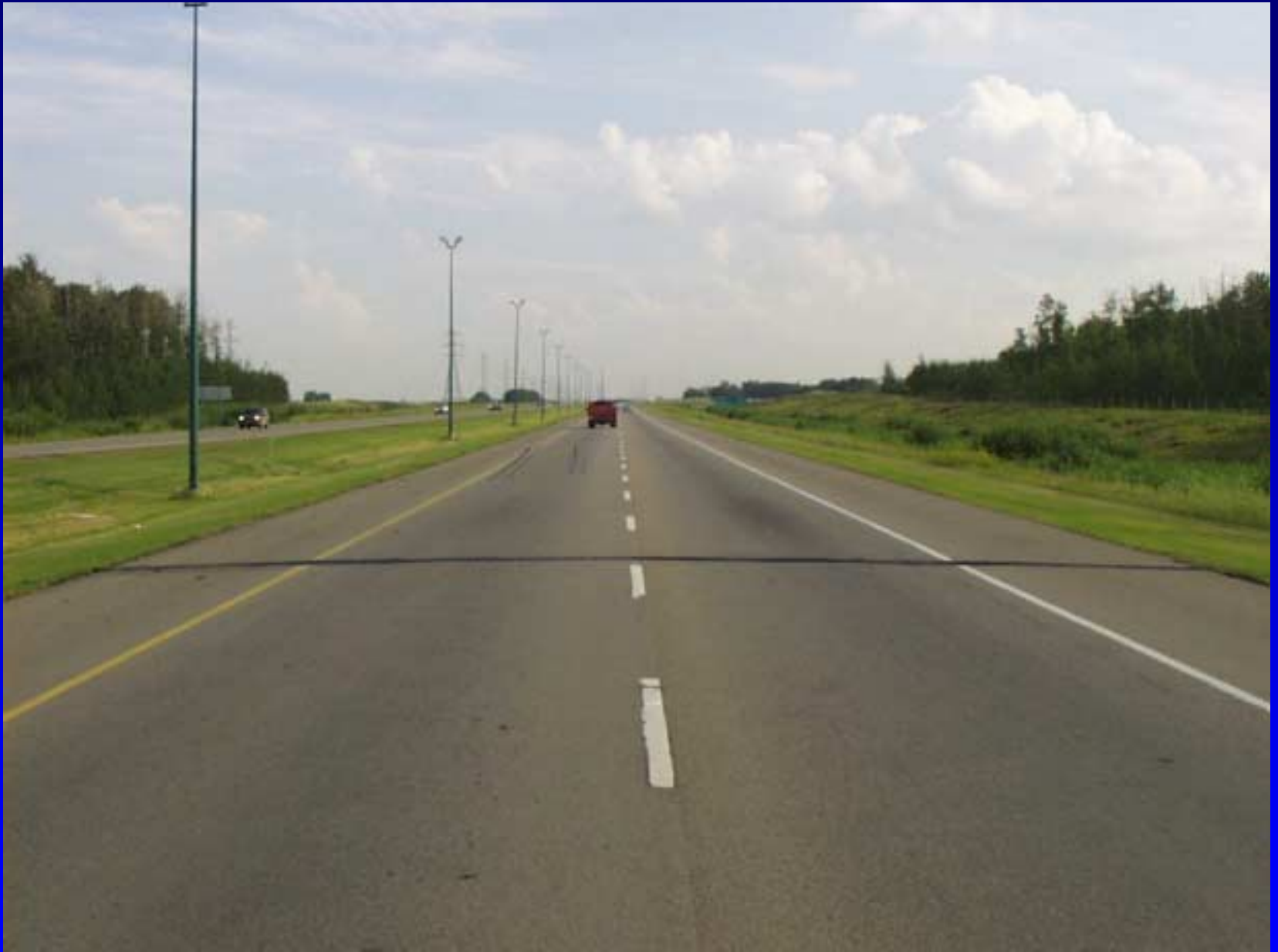
Styrofoam Installation, Edmonton, Alberta
