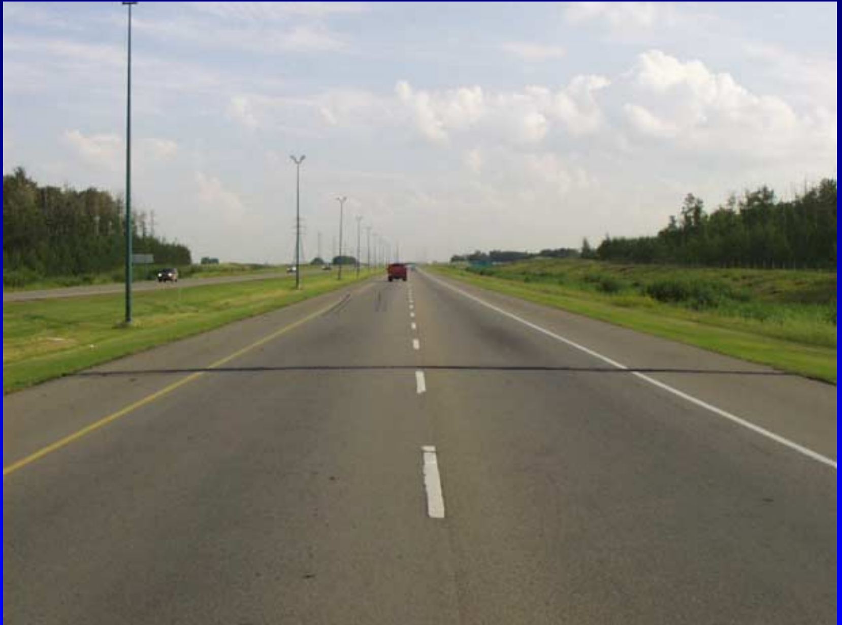
Styrofoam Installation, Edmonton, Alberta
