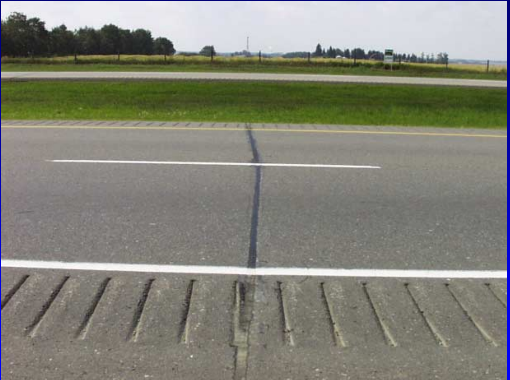
Saw and Seal, South of Edmonton, Alberta
