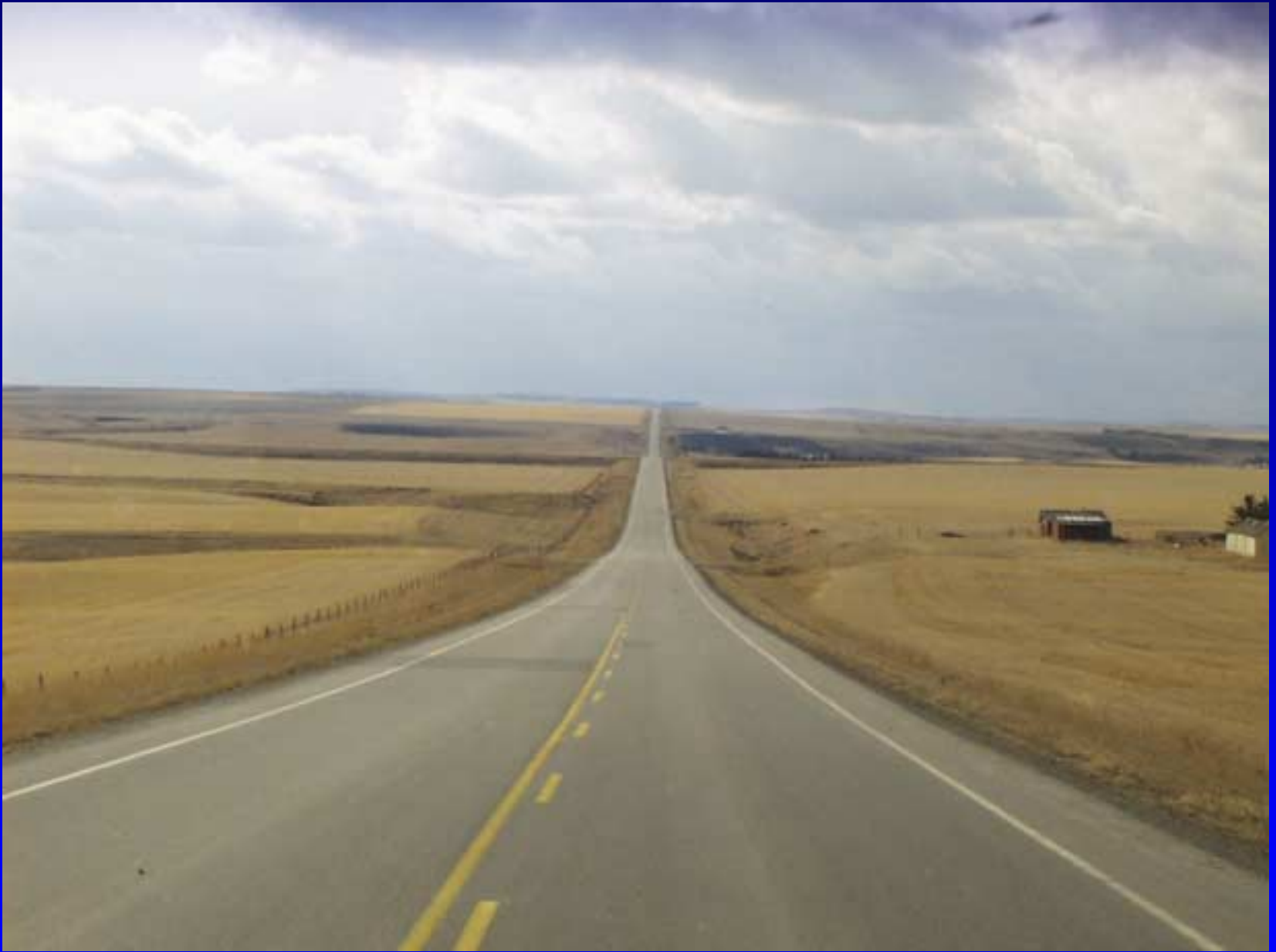
Secondary Highway, East of Calgary
