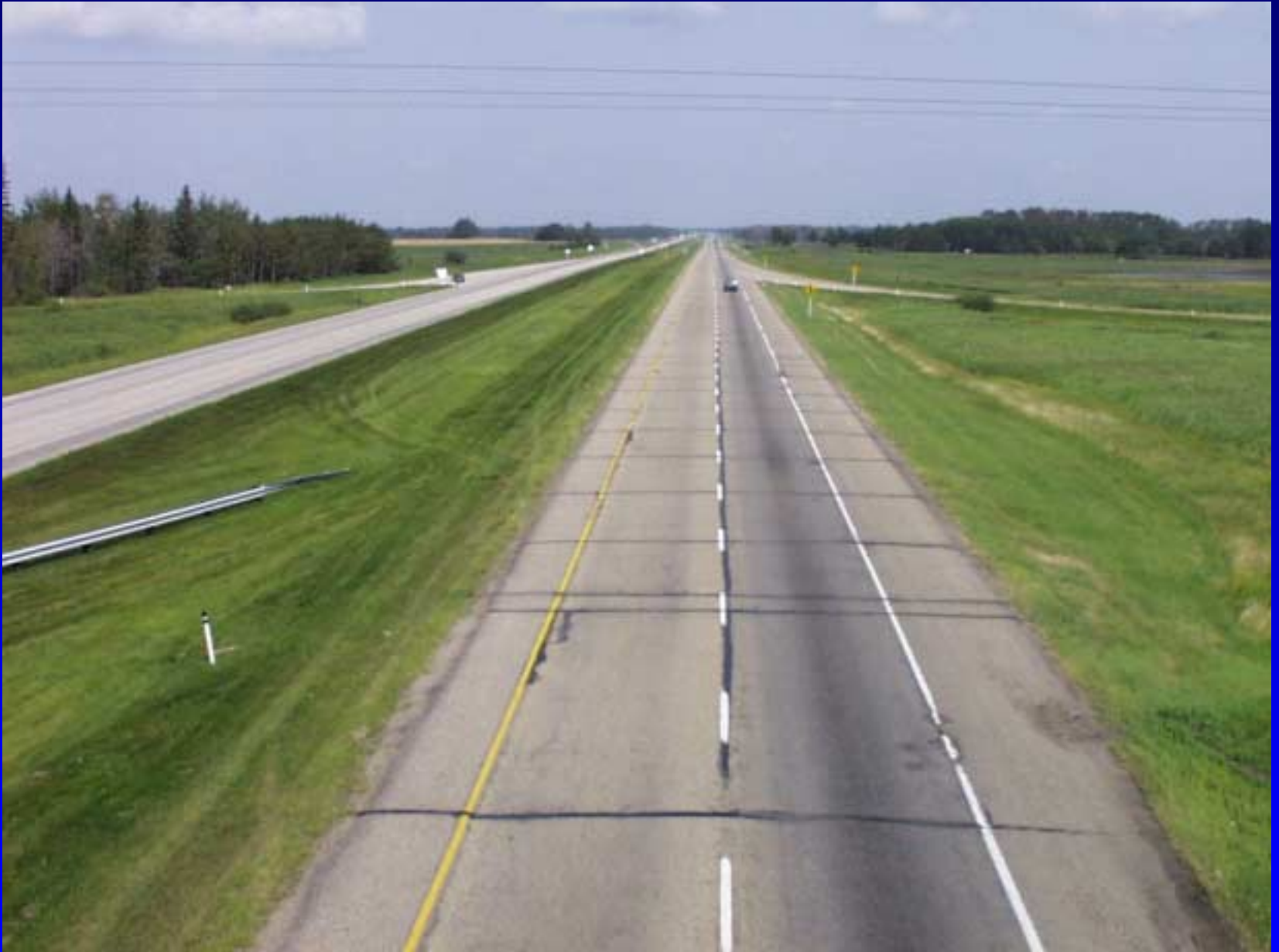
Hwy 2, South of Edmonton, Alberta
