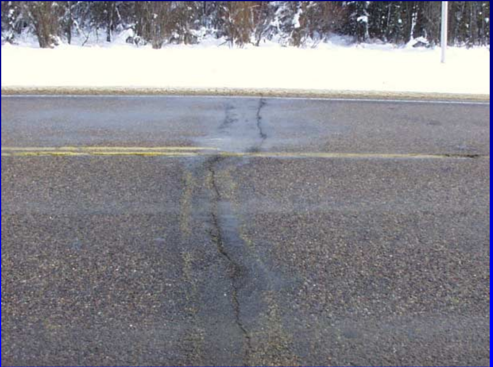
Spray Patch in Foreground, Cold Mill and Inlay in Background
